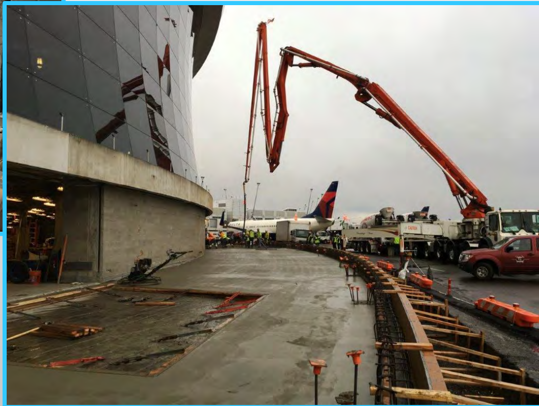
Rebar installation and concrete pour for CT building extension
